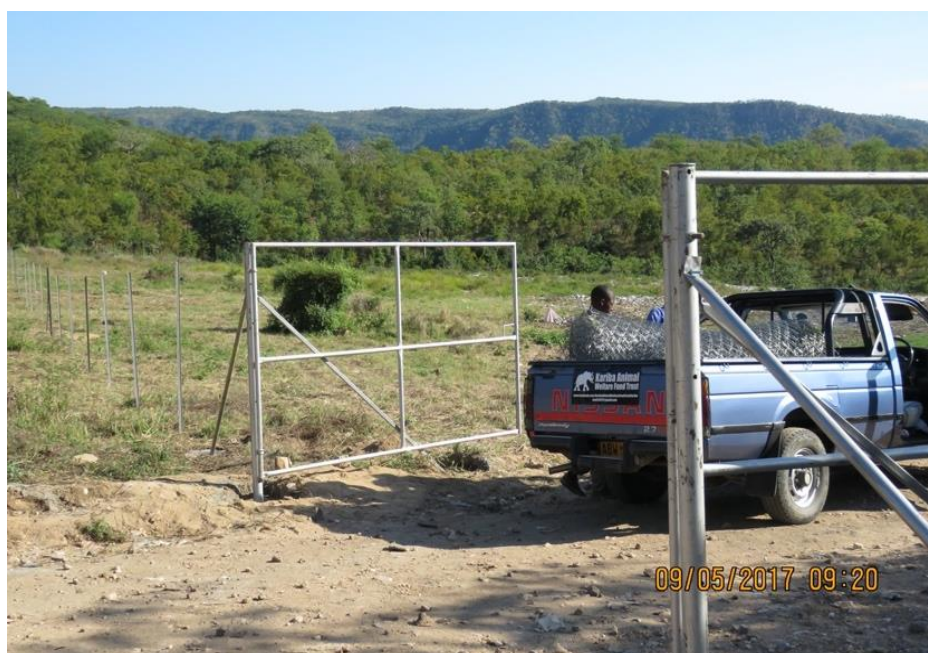
The fence around Kariba Rubbish Dump. Photo by KAWFT
